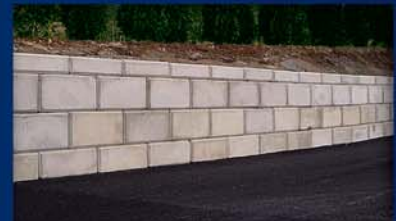
2' x 1' x 4' Interlocking Cap, 1100 lbs. 2' x 2' x 4' Interlocking Plain Block, 2200 lbs.
